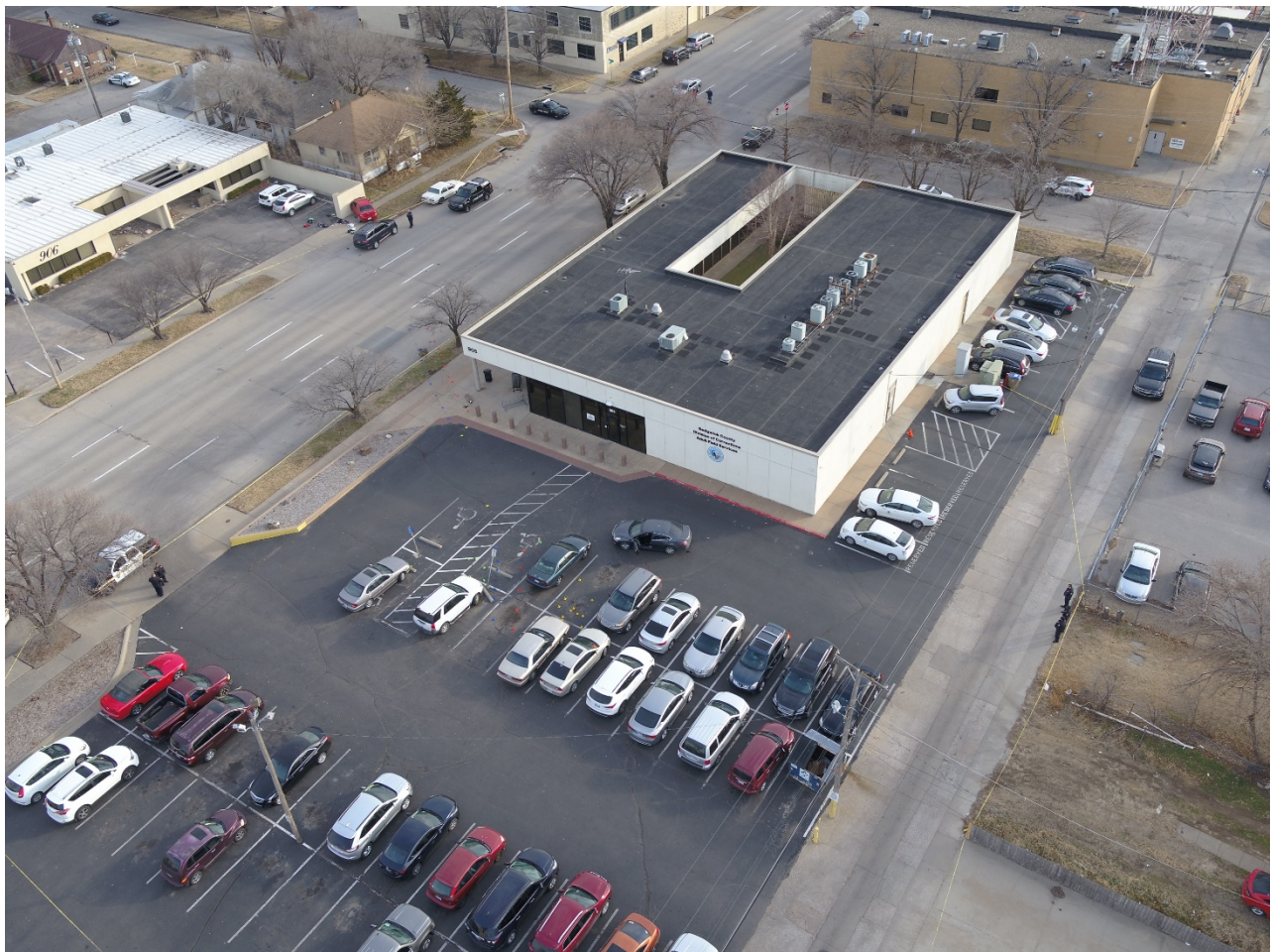
Aerial of 905 N. Main following shooting.
